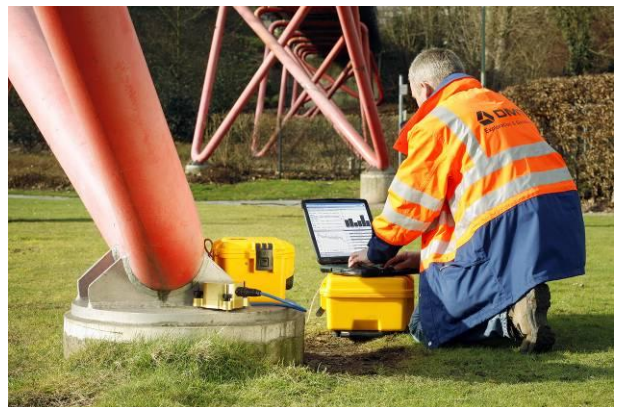
Monitoring of footings
