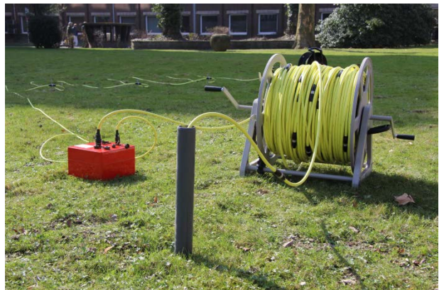
Borehole cable with decoder box
