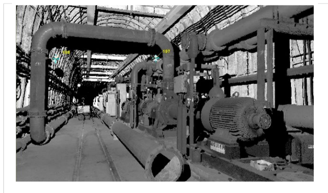
Point cloud of a pumping station in an underground coal mine
