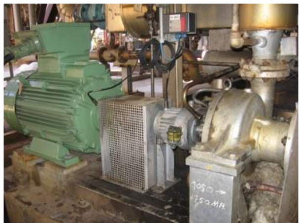
Centrifugal pump 1P451B Ruhrpumpen SVN-4X13
