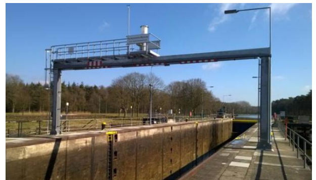
Totalstation on bridge
