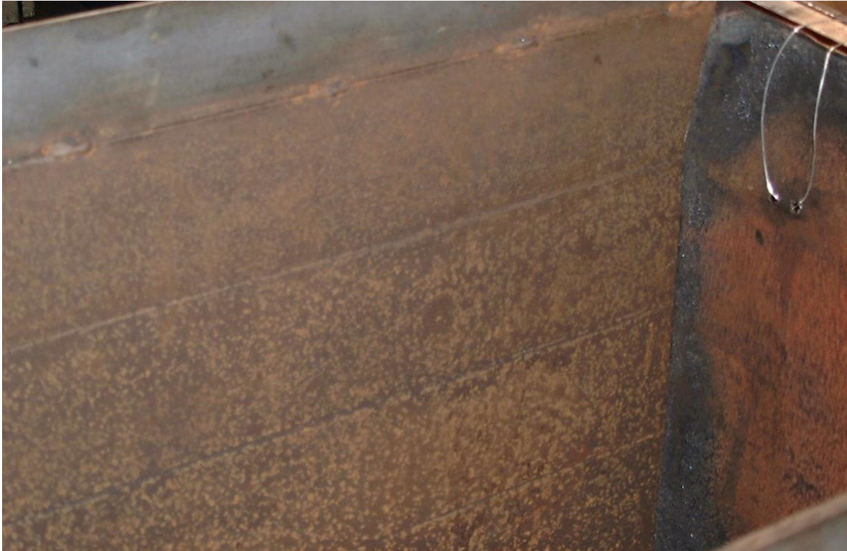
Figure 5: Marking lines for the individual layers in the stamping box
