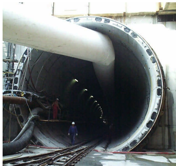
Application in tunneling
