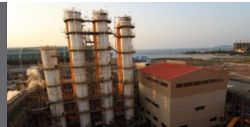
Scrubber Area and Gas Exhauster Unit
