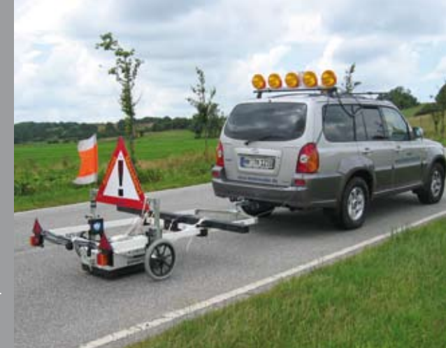
Investigation and localisation of road setup and components via ground penetrating radar"
