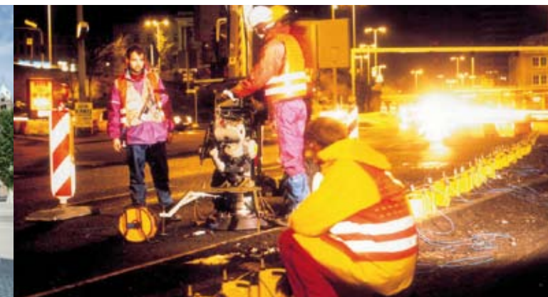
Sewage line examination in Wuppertal
