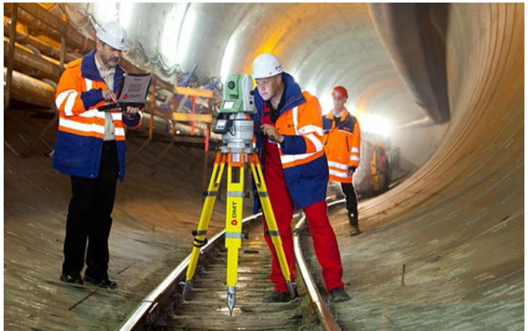
Tunnel survey with GYROMAT 3000
