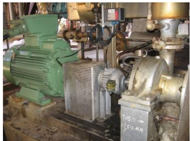
Centrifugal pump 1P451B Ruhrpumpen SVN-4X13
