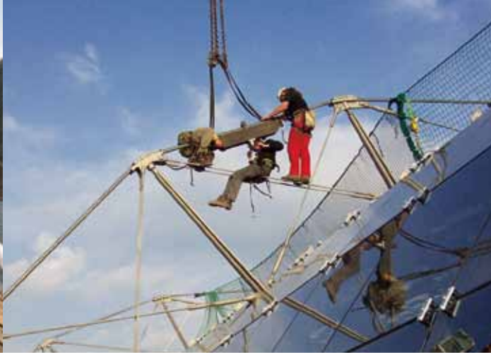
Measuring rope tension at Lehrter Station, Berlin
