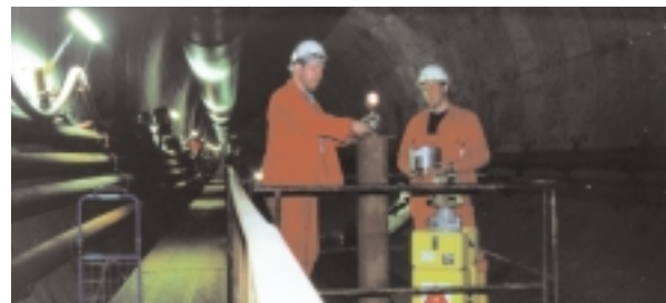
Surveying work in the tunnel
