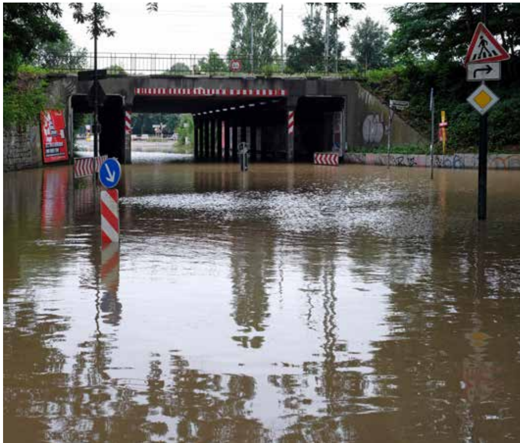
Roads and bridges were also damaged by the flooding in Germany
